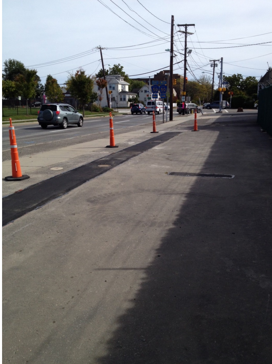
Restored trench at 60/66 North Clinton Avenue adjacent to Clinton Avenue
