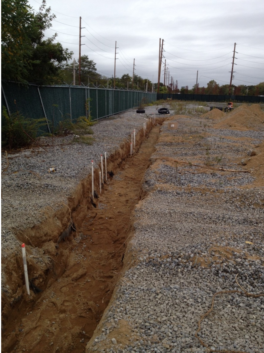
Excavated trench at OU-1 North
